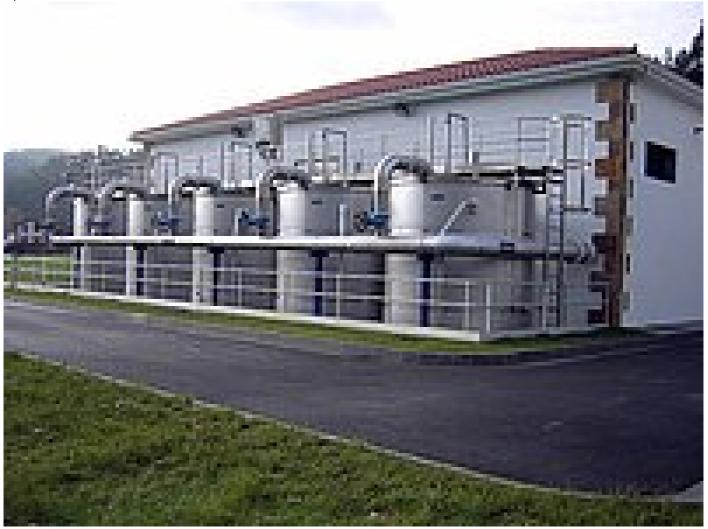
Effluent filtration serves for increased removal of suspended solids (SS), BOD, COD, phosphorus (P) and nitrogen (N). About 20 % of German effluent is filtered.
