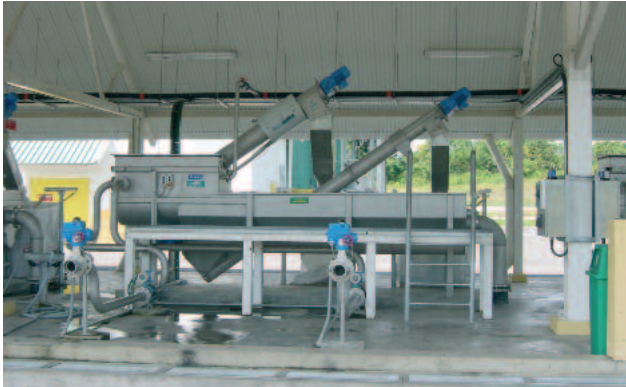
ROTAMAT® Sludge Receiving Station with grit trap and grit classifying screw
