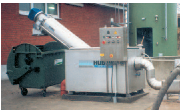
Outdoor installation of a ROTAMAT® Ro 3.1 Septage Receiving Station with frost protection
