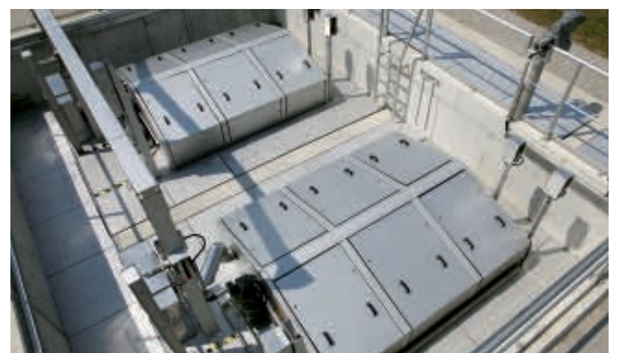
HUBER RoDisc® Rotary Mesh screen installed in a concrete tank
