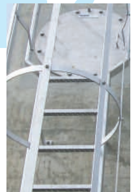
Safety access ladder with fall arrestor and manhole cover set in concrete
