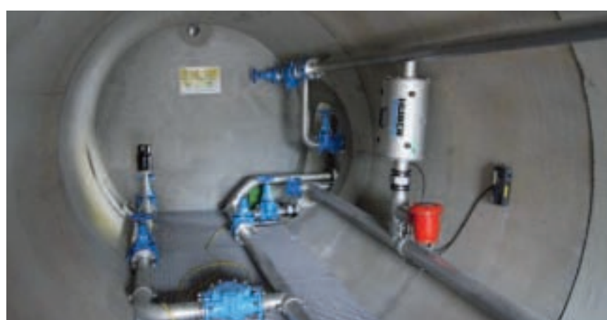
Valve chamber with air filter plant L251 after installation
