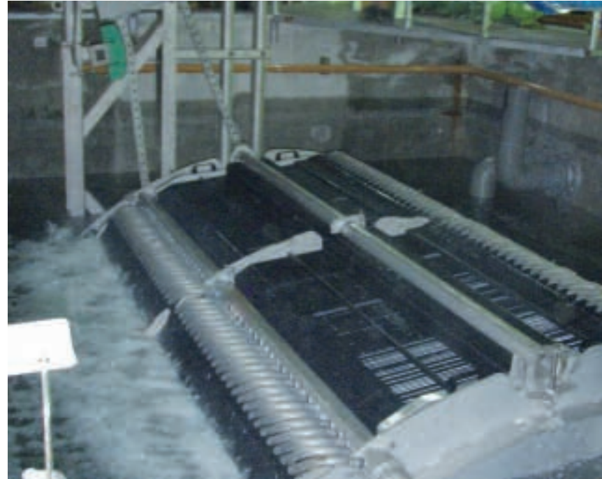
HUBER VacuumRotationMembrane VRM® Bioreactor
