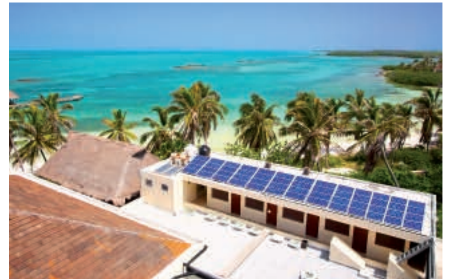
More and more hotels install sustainable power and wastewater systems
