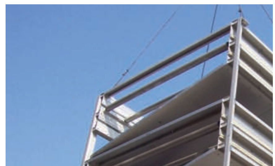
Line 3 during installation
