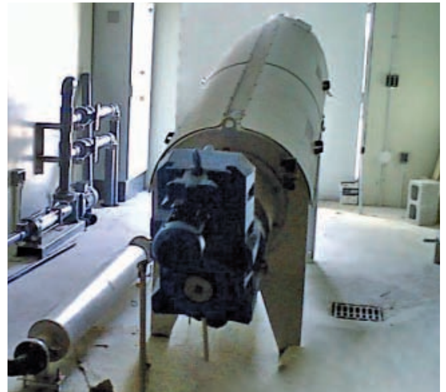
ROTAMAT® Screw Press RoS 3Q installation on the Caribbean Islands
