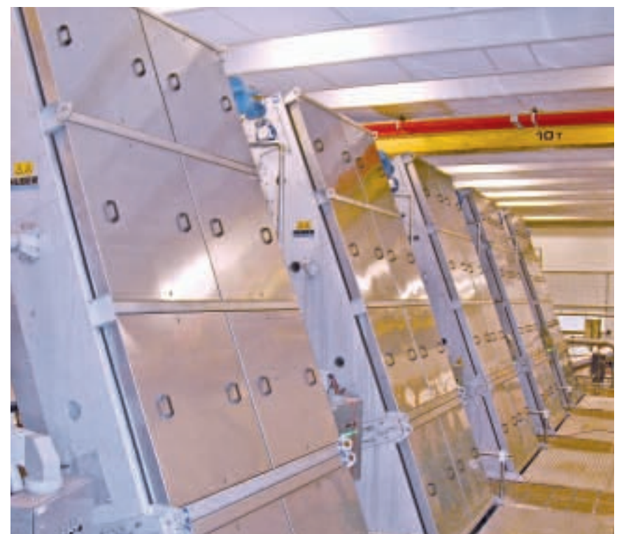
HUBER Belt Screen EscaMax® on WWTP Lynetten
