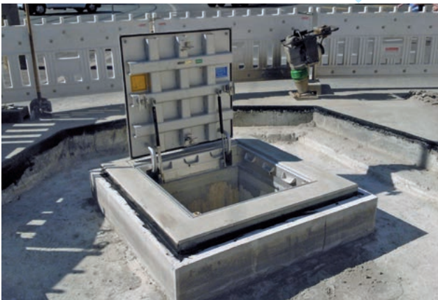
SD7 during installation
