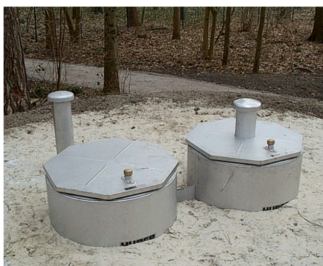
FSG 1 Prefabricated manhole installation
