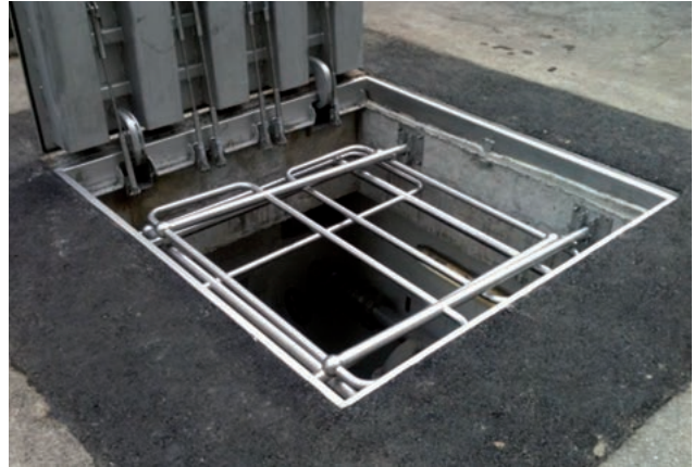
SD7, open cover, folded down railing
