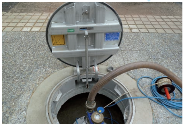
Manhole cover SD7.R, round design, class D400
