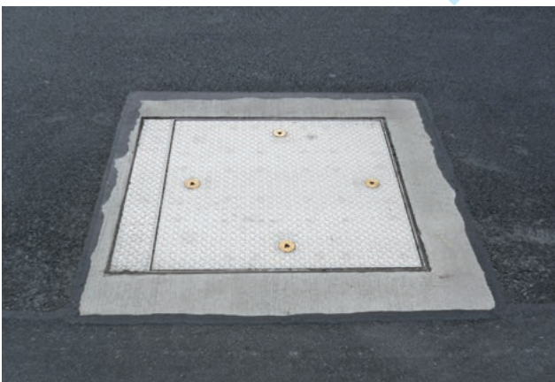
SD7 after installation into the driveway
