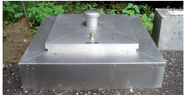
SD 1 Rectangular manhole cover with crown cover
