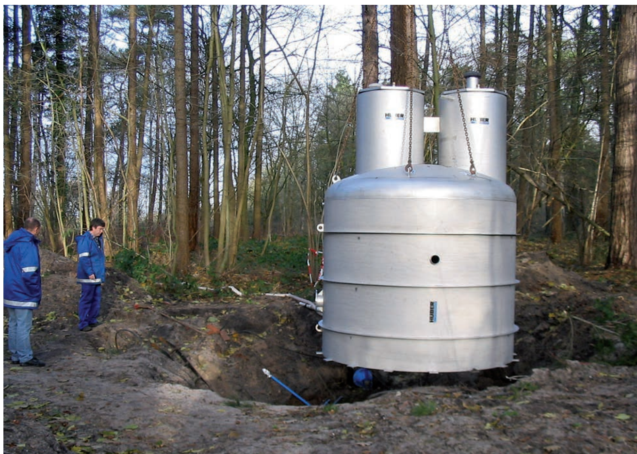
FSG 1 Prefabricated manhole during installation
