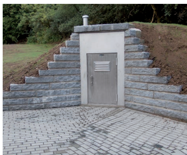
FSG 1 Prefabricated manhole with entrance door type TT2.1
