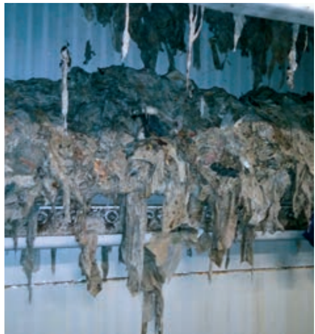
Figure 3: High pollution load on a rake bar.
