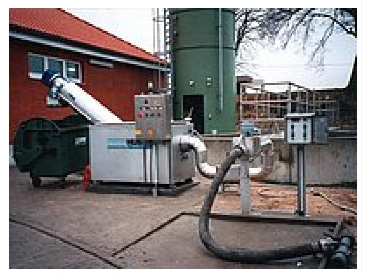
Well-proven, efficient and rugged Septage Receiving Station
