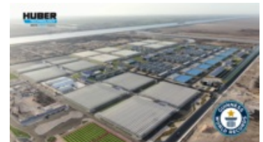
Aerial photo of the Bahr El-Baqar plant ; © Orascom Construction PLC and The Arab Contractors
