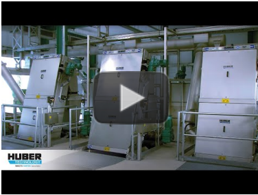
Video: RakeMax® Multi-Rake Bar Screen for mechanical preliminary wastewater treatment at a municipal WWTP
