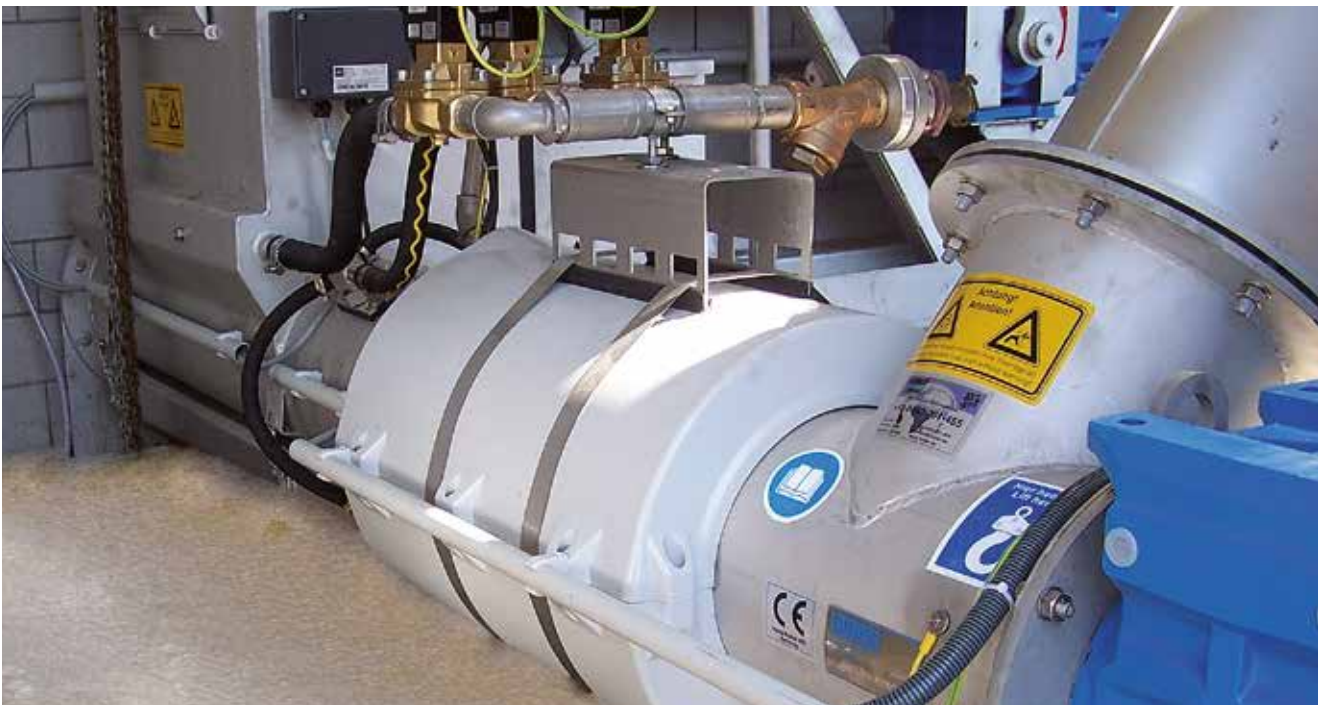
HUBER Screenings Compactor Ro7 – compact design, with optional screenings washing.
