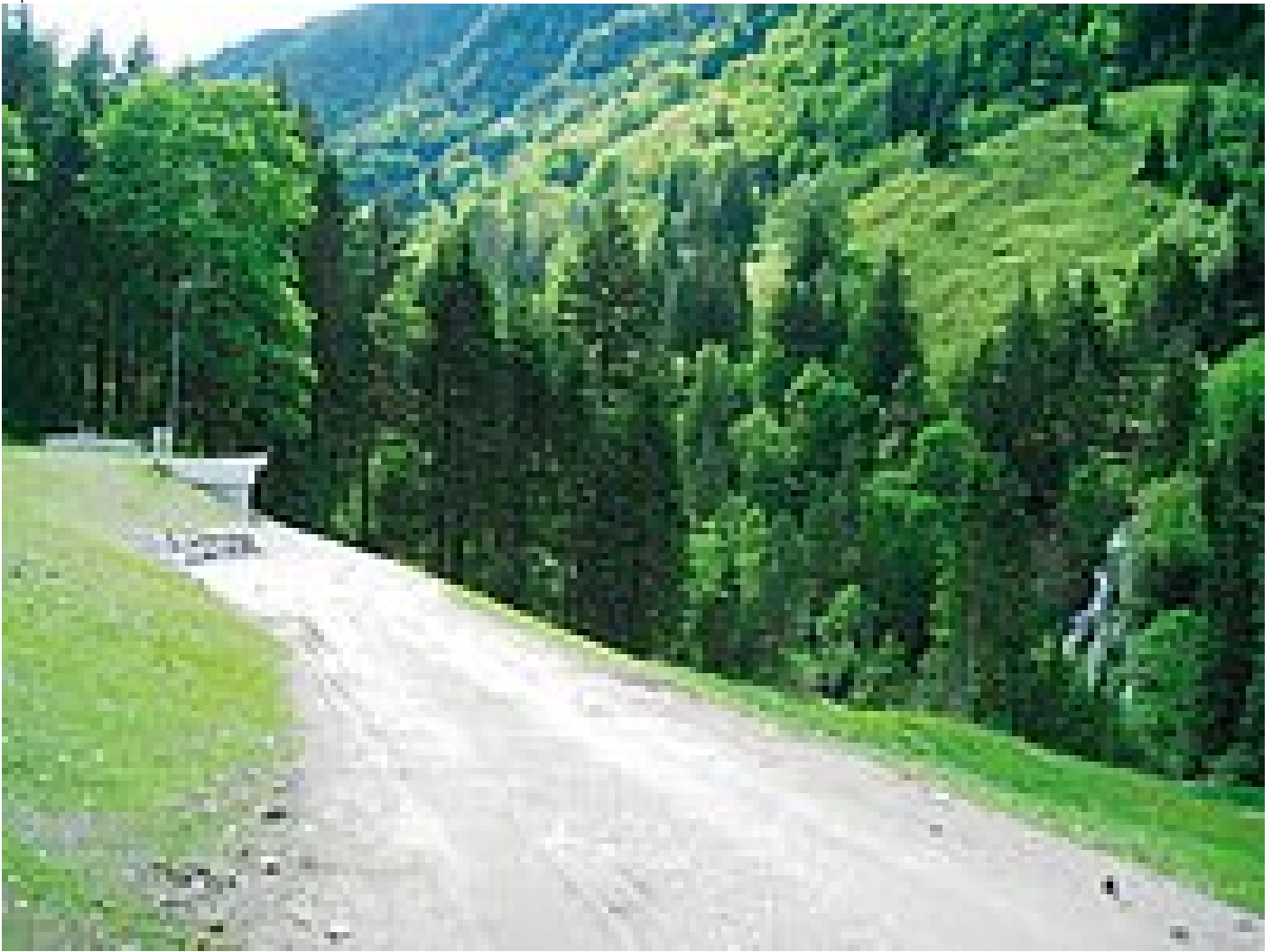
The inlet structure on the left, the spring overflow on the right
